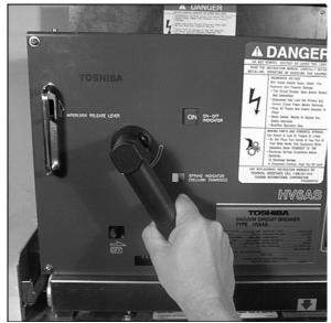
Fig. 26 Manually Charging Breaker
